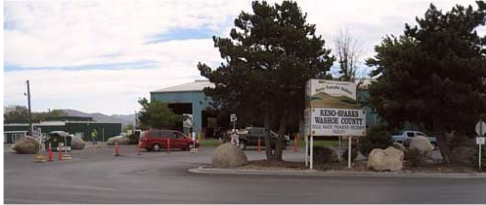
Sage Street Transfer Station, Reno
