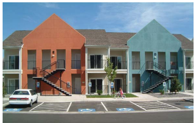
Affordable Housing Development, Reno, Nevada
