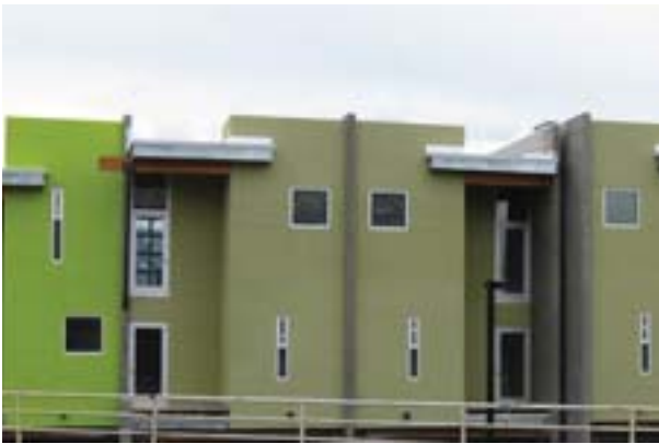
Eight on Center - one mile from downtown Reno
